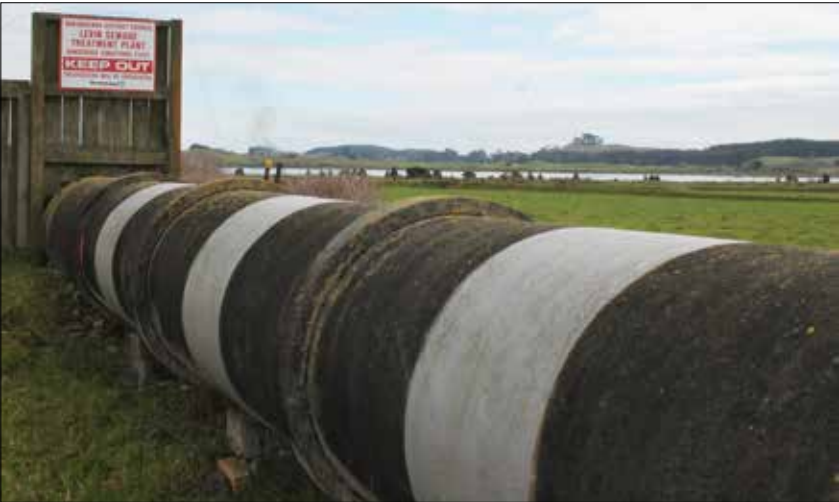
The old concrete sewage pipe that will be replaced at the Mako Mako Road treatment plant.
